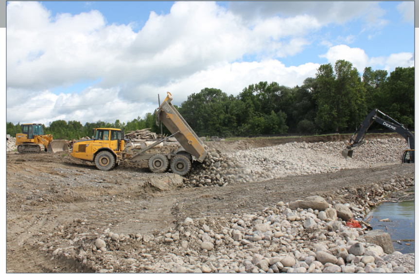
Figure 28: Construction of the marina basin at Friday Harbour. (Geranium Corporation, 2012)
