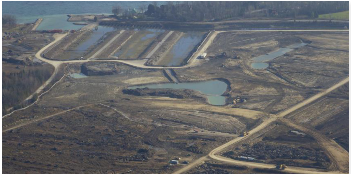
Figure 29: Tree removal and site preparation work for the Marina Village at Friday Harbour. (Save Lake Simcoe, 2012)
